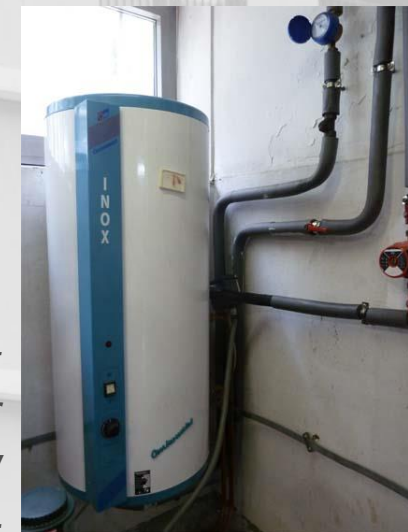
Indirectly heated hot water storage heater of nominal capacity 120 L
