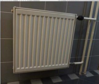
Vertical exposed and Panel radiators in concealed two-pipe fan coil sanitary facilities units
