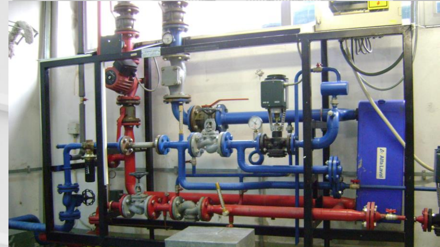
Indirect type of district heating substation in the basement of the nominal heat power 250 kW (manufacture date 2000.)
