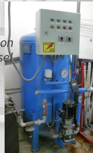
Indirect type of district heating substation in the basement of the nominal heat power 250 kW (manufacture date 2000.)
